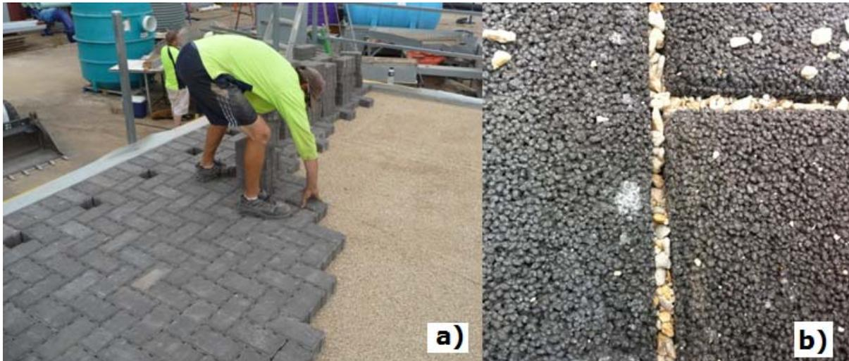
Figure 5. (a) Herringbone Pattern Installation, (b) Bedding Aggregate in Paving Joints
