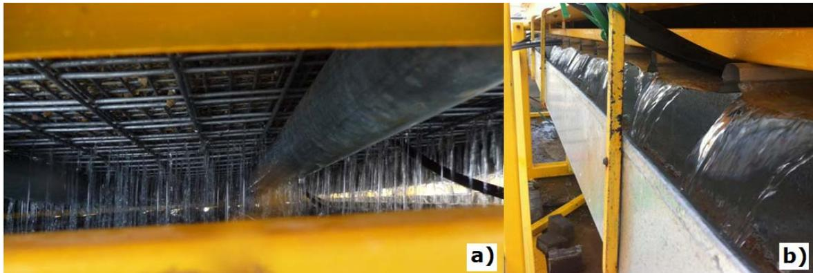
Figure 3. Water Infiltrating through Pavement Structure (a) into Drainage Gutter (b)
