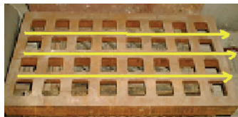
Figure 9 – Problems associated to the hydraulic design of the macro-grate 1.
