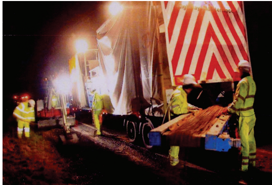
Figure 2. StoneMaster® in Action on Motorway.
